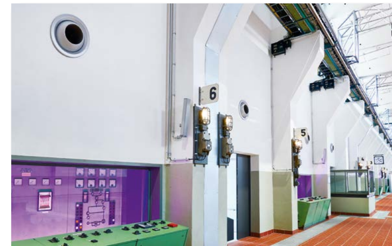
Adjustable jet nozzles are ideal for supplying air to this very large hall.
